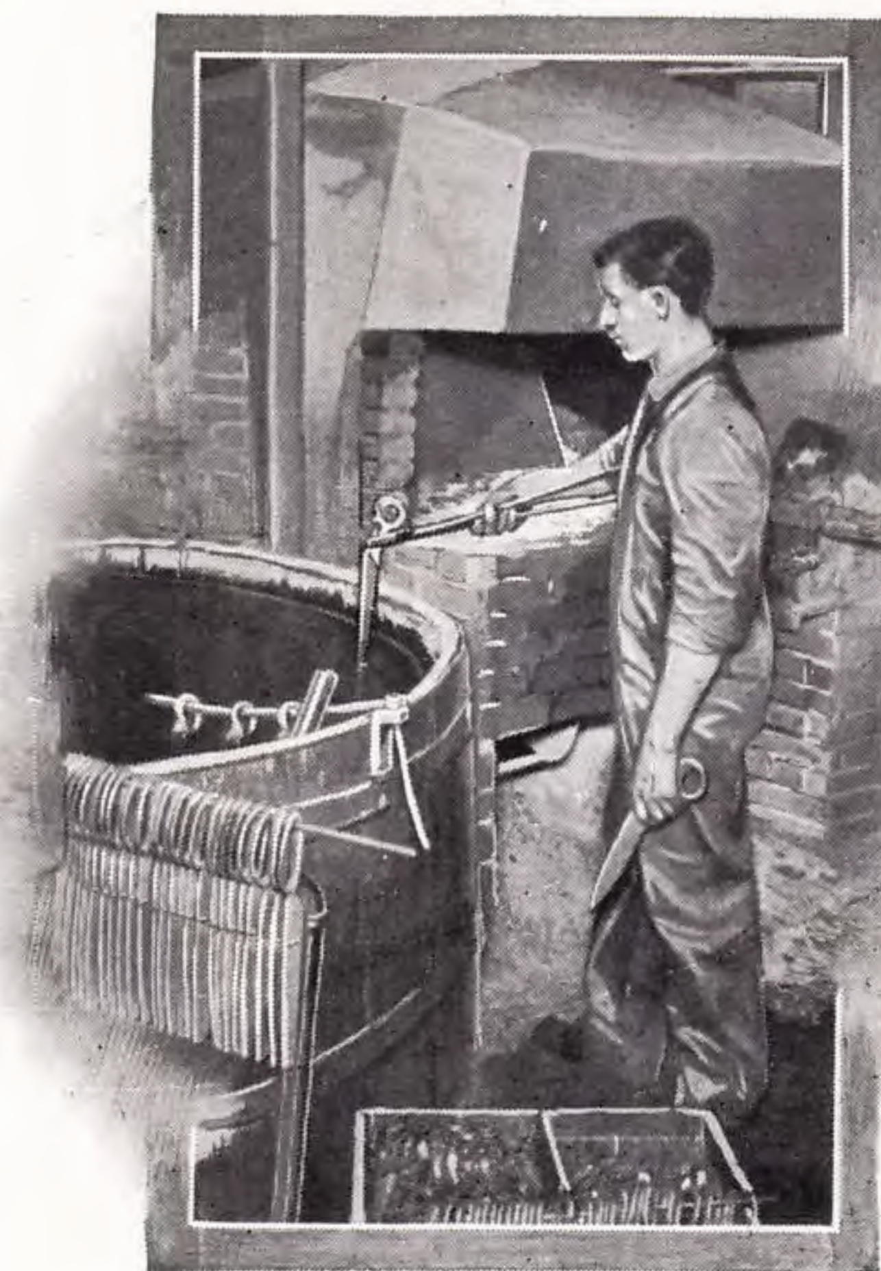
'Hardening the Wiss Shear Blade'
