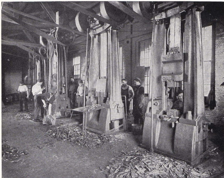
Wiss Forging Department where the frames of Wiss Shears are forged under powerful drop-hammers
