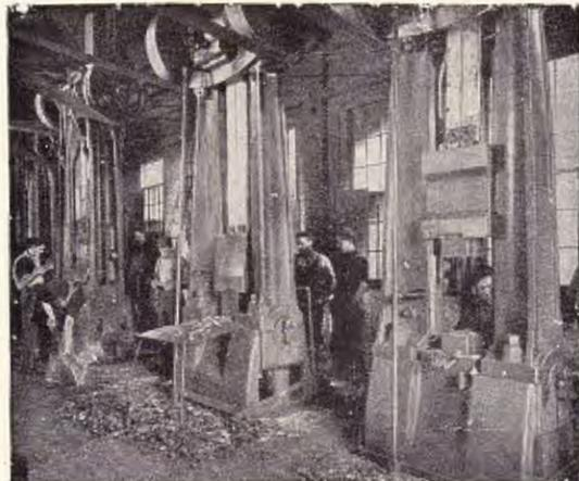
WISS Forging Department, where the frames of WISS Shears are forged under heavy drop hammers
